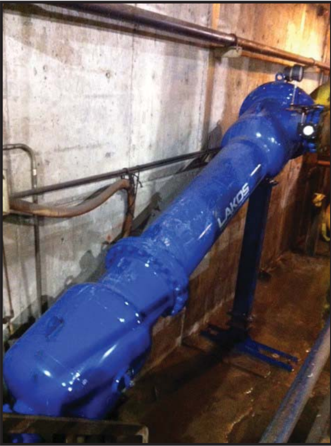
The JSK-2650-L/LFG industrial separator has a flow rate of 2650 - 4900 GPM
