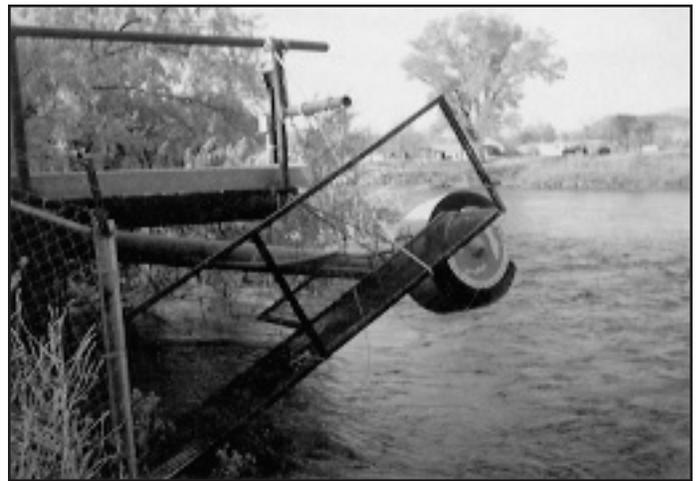
*Pumping 640 U.S. gpm (145 m<sup>3</sup>/hr) at 90 psi (630 kPa), this pump station in Wyoming relies on a PLUM CREEK Screen to prevent organics and debris from interrupting water service to its customers. A galvanized steel shield has been added for protection against large or heavy objects carried by the river's swift current. Note the shield's notched side-opening that allows PLUM CREEK's backwash jets to blow away particles attracted to the screen.*
