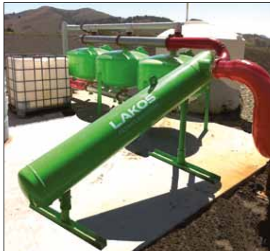
BRS- Backwash Reduction System
