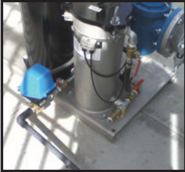
TowerClean System with the best of both worlds: a Solids Recovery Vessel (SRV) that offers zero liquid loss, and an Automated Ball Valve (ABV) for maintenance free purging.
