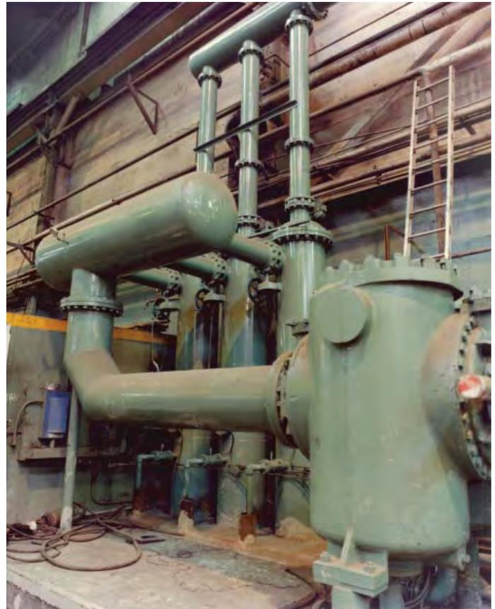
*Three vertical profile LAKOS RFD Separators at work in the plate mill.*
