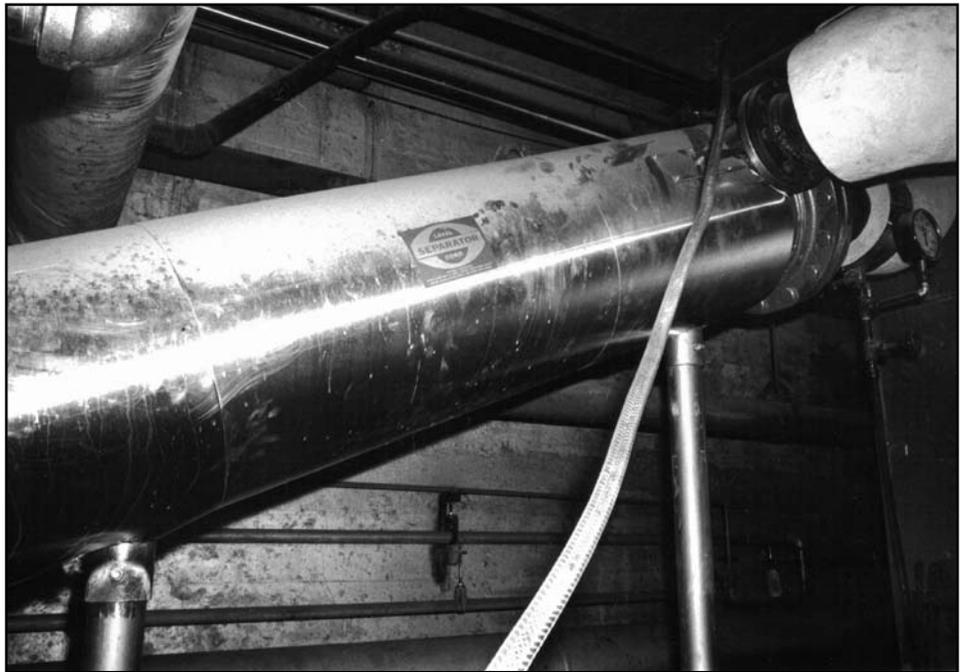
*This 8" Lakos Industrial Separator with a flanged dome has been covered with an insulating material as 180° condensate water is passed through the separator to remove troublesome solids before the water enters a polishing filter.*
